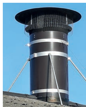
Vent stacks secured against birds.
